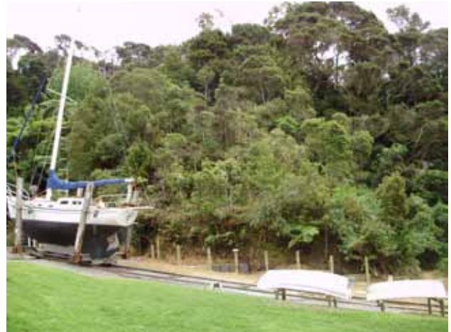
Boat slipway showing unconsented wall to hide infrastructure on esplanade reserve land. Cuts to bank and removal of bush visible. Note: two dinghy racks on the reserve.
