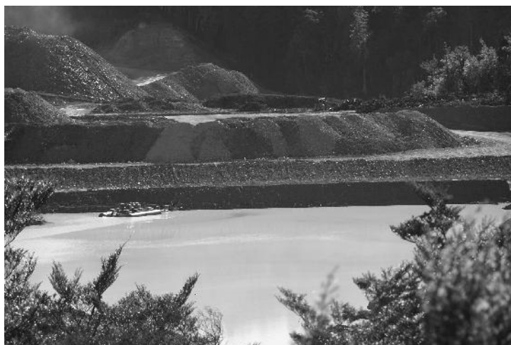
Oceana Gold rock dump and tailings dam, Victoria Conservation Park, near Reefton on the West Coast of the South Island.
