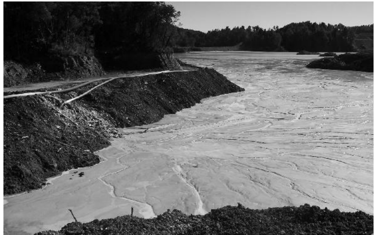
Oceana Gold tailings dam in Victoria Conservation Park. In order to extract the gold the ore is ground to the consistency of toothpaste and tailings and waste rock are dumped in valleys adjacent to the mine.
