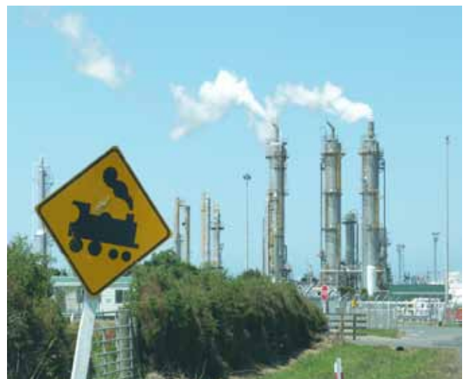
Fig 4 - Kapuni Production Station
