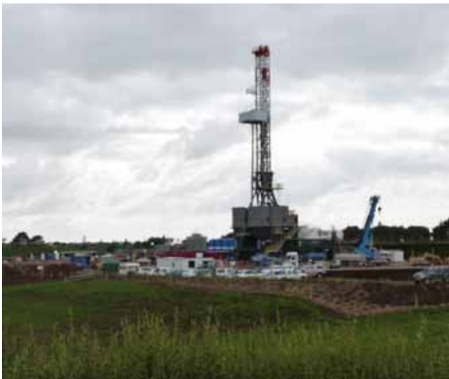
Fig 1- Todd Energy's Mangahewa E well site in North Taranaki
