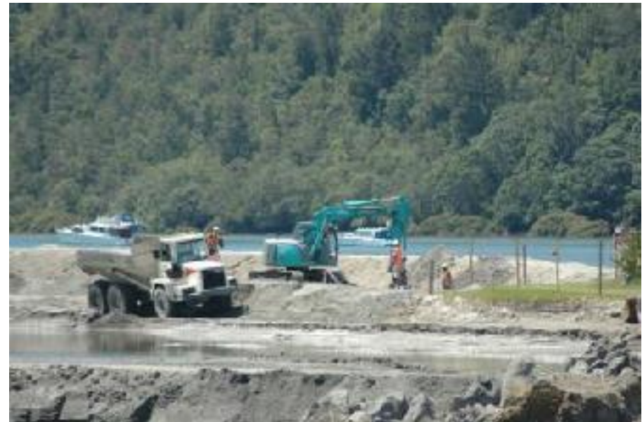
Construction of Whangamata Marina
